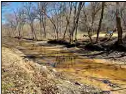
Accumulated sediment within the C&O Canal prism upstream of Lock 20 that will be removed.
